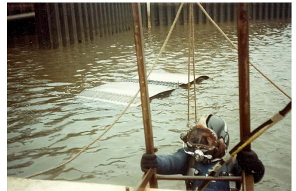
Diver Scott Anderson, of Logan Diving & Salvage, entering the water to install a 36" three piece extended range clamp on a failed pipeline in Georgia's Savannah River.
