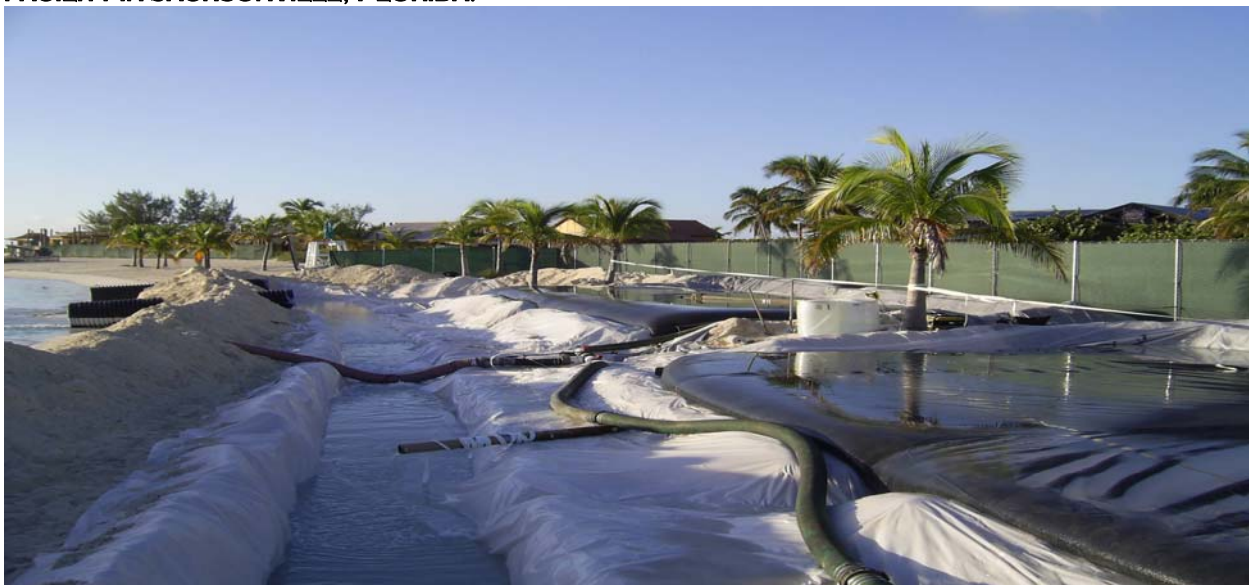
GEO TUBE SPOIL AREA STATION FOR SUBAQUEOUS SEDIMENT CONTAINMENT
